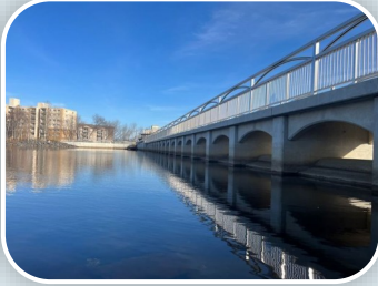
Bridge Panels Manufactured by Miller Precast Ltd.
